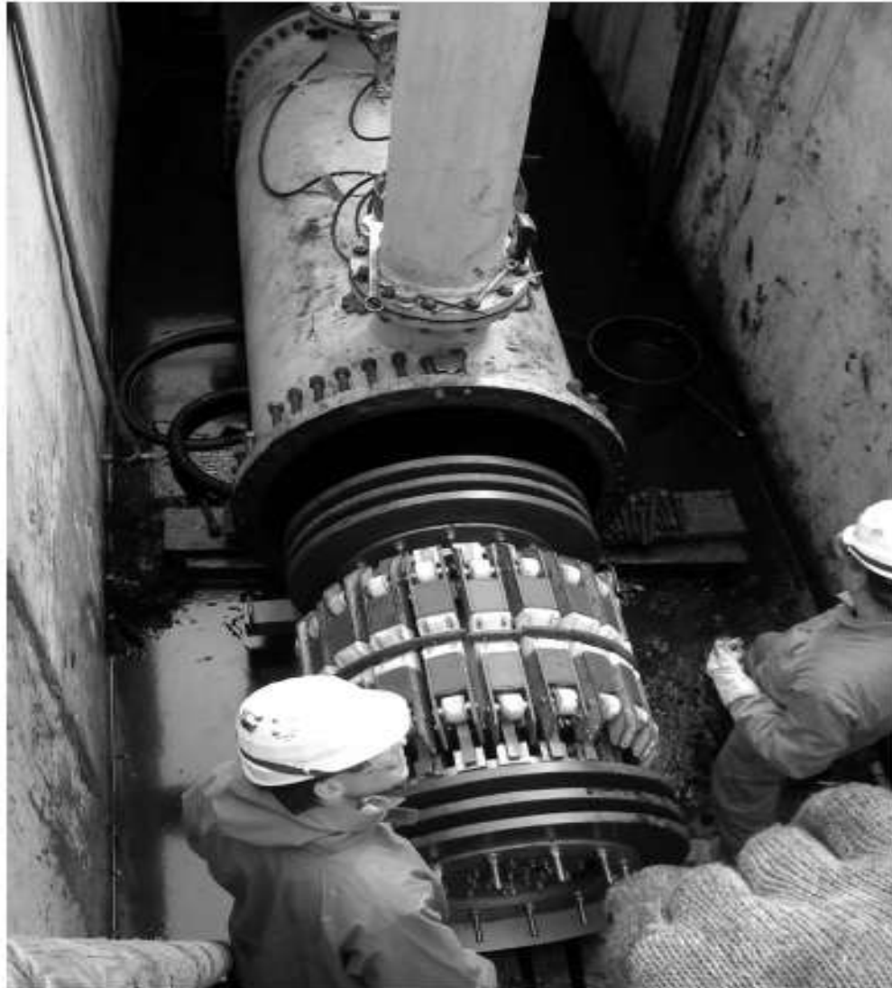
Figure 5: Manoeuvring the Magnetic Flux Leakage Pig into the Pipeline
